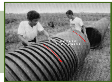
3.) Rotate clockwise the coupling into the spigot until reaching the checkmark.
