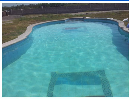
Water Purification Pools at the Water Works
